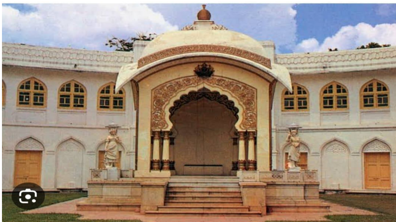
Jubilee Hall and Pavilion
