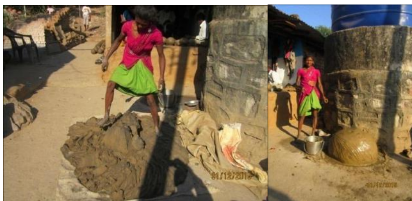
Fig. 3a: Kneading the mud
