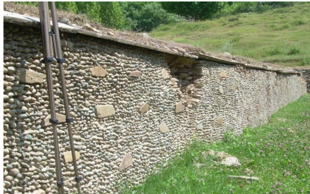
Fig.4: Pebble style wall of a monastery at Harwan (Lower terrace).
