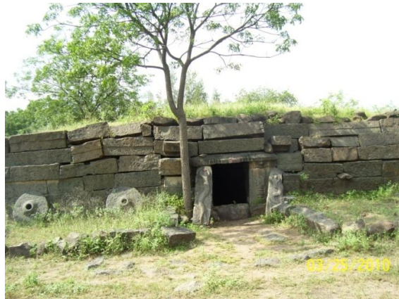
Plate 1 Picture shows front view of Mahadev Temple.
