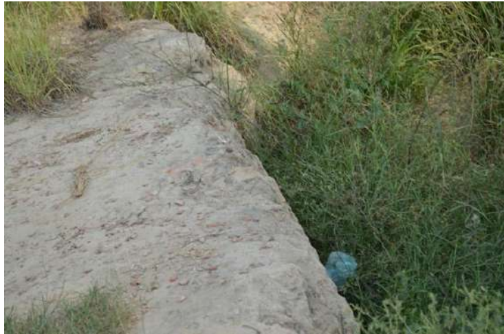
General View of Hans Dahar
