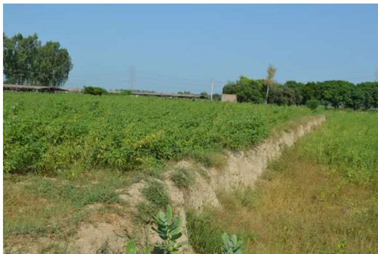
General View of Kalwan-1
