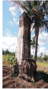
16. b. Water Tower
